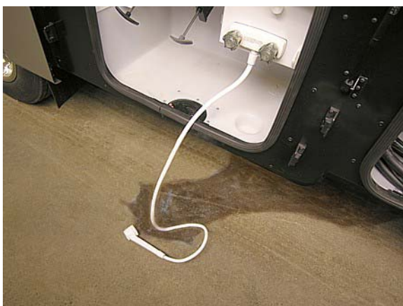
Using exterior shower to drain waterline (Typical view - appearance on your coach may differ)
