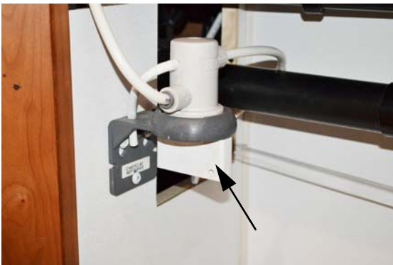
Diverter Plug (installed in filter socket)
