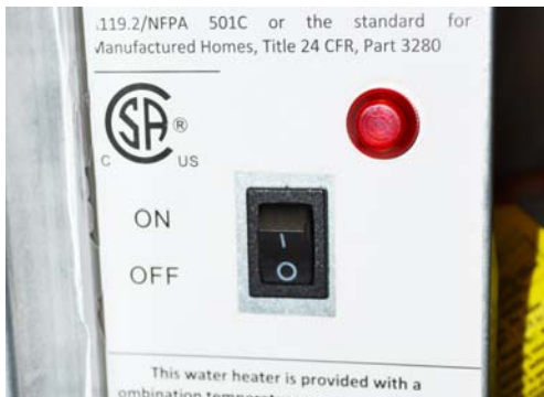
Water Heater (Tankless) Power Switch
