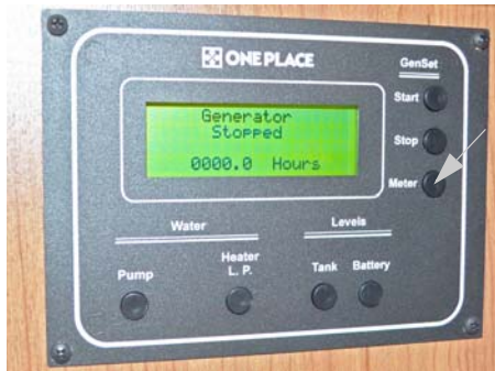
Generator Hourmeter Button -Typical View
