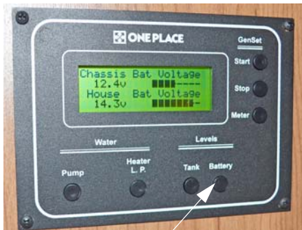
Battery Levels Switch
