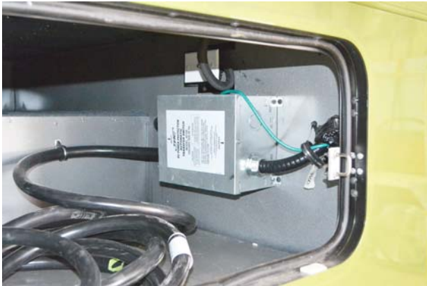
Automatic Power Transfer Box (Located inside or behind utility compartment) -Typical installation shown
