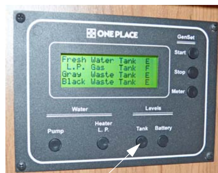
Tank Levels Switch
