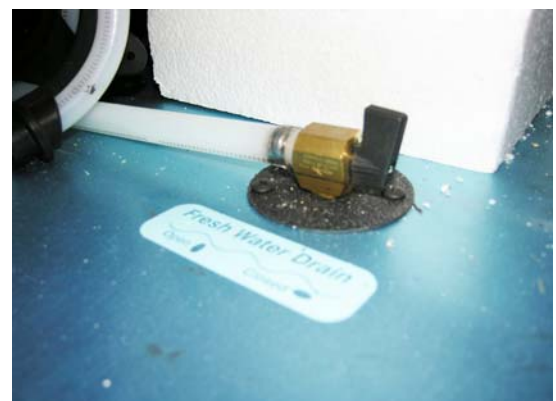
Water Tank Drain Valve - Typical Installation
