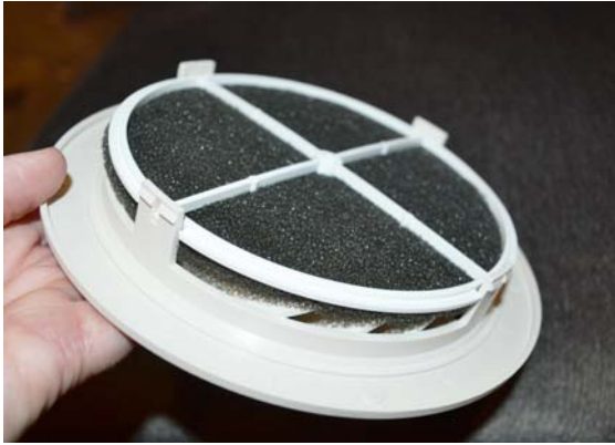
Air Filter (Located on back side of Return Air Vent) -Typical View
