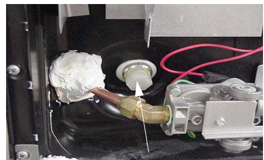
Water Heater Drain Plug (Remove with socket)
