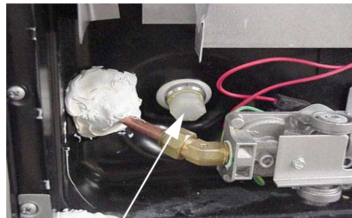
Water Heater Drain Plug (Remove with socket)
