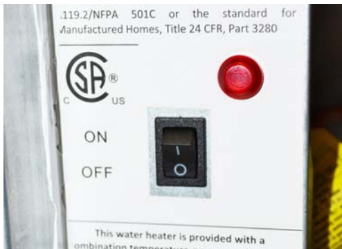
Water Heater (Tankless) Power Switch -If Equipped
