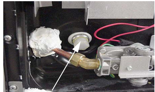
Water Heater Drain Plug (Remove with socket)
