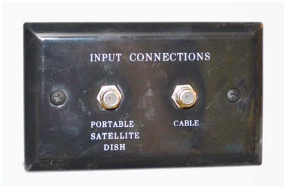
Cable TV and Satellite Dish Connections (Located in utility compartment)
