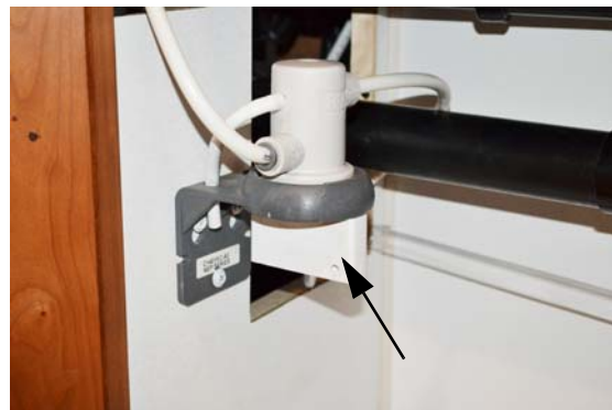
Diverter Plug (installed in filter socket)
