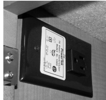
Front TV Ignition Switch Interlock -Typical View
