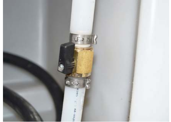
Water Tank Drain Valve -Typical installation shown
