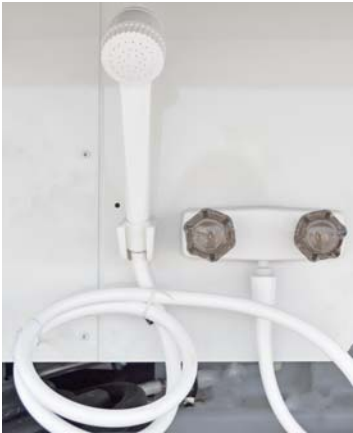
Exterior Shower/Wash Station -Typical View
