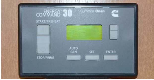
AGS Control Pad (Located near monitor panel)
