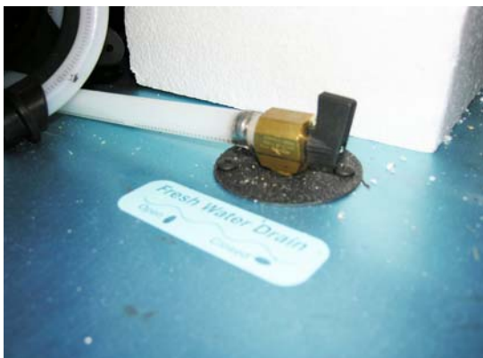
Water Tank Drain Valve - Typical Installation
