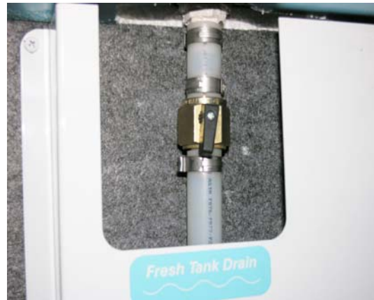
Water Tank Drain Valve - Typical Installation
