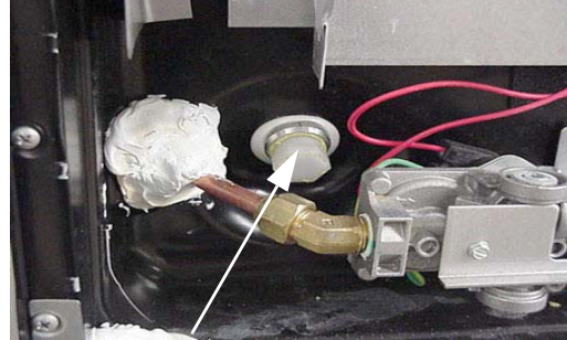
Water Heater Drain Plug (Remove with socket)
