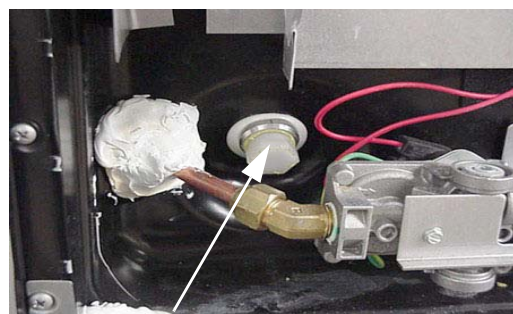
Water Heater Drain Plug (Remove with socket)
