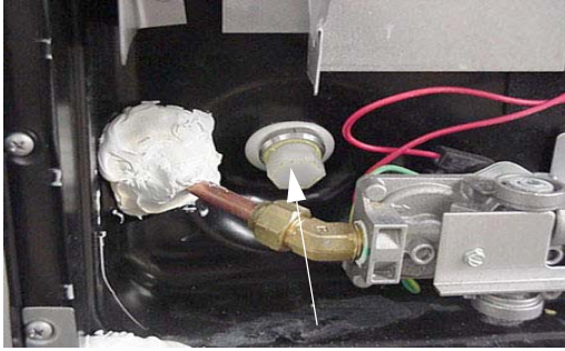
Water Heater Drain Plug (Remove with socket)
