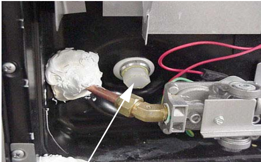
Water Heater Drain Plug (Remove with socket)
