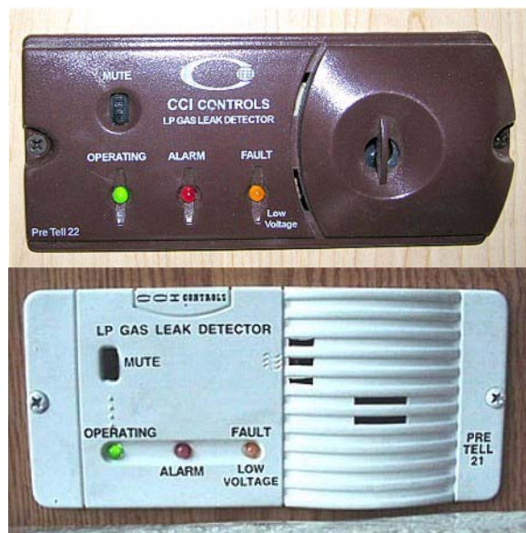
Propane Gas Leak Detectors (Typical)
