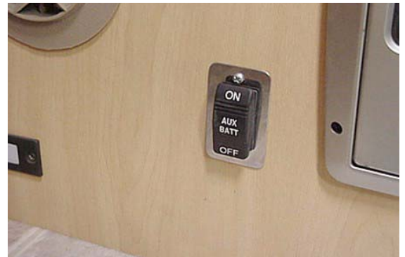
Aux. Batt. Switch - typical (Near entrance door)
