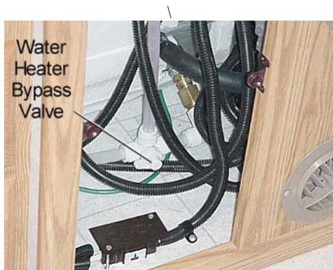
typical installation
