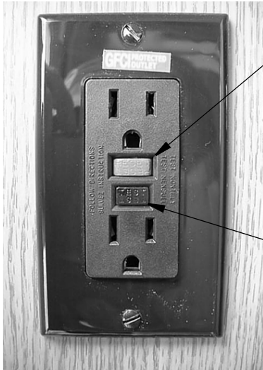
GFCI Outlet (Ground Fault Protector)
