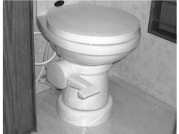
2. To flush the toilet, push the lever all the way down until sewage leaves the toilet and bowl is rinsed clean.
