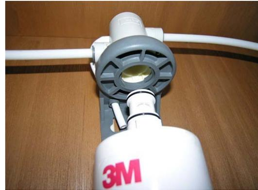
Insert new filter up into filter socket
