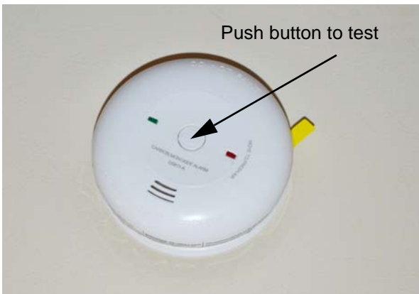
Carbon Monoxide Alarm
