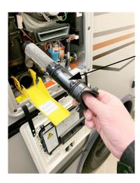
Water inlet filter pulled out and removed.
