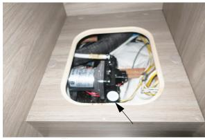
The water pump strainer is located closest to the inside
