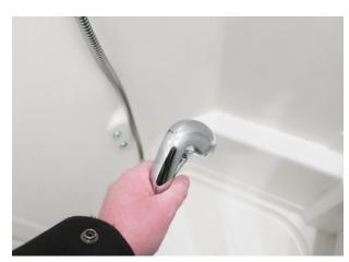
Point shower head at the drain and squeeze until water stops flowing.
