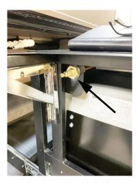
Located under the sink table is the attachment for an LP tank that will run the stove.
