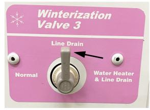
Winterization valve in the "Line drain" position.
