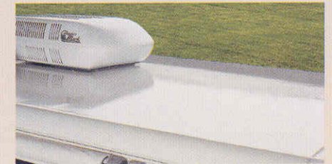
One-year-old Winnebago Industries fiberglass roof
